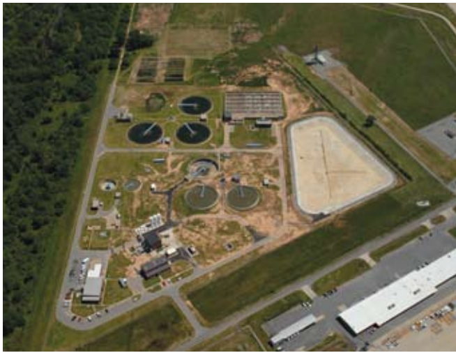
Adams Field Wastewater Treatment Facility
