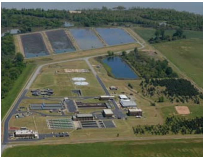
Fourche Creek Wastewater Treatment Facility
